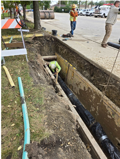
Acqua Contractors Corp. pulling water main pipe through directionally drilled holes
