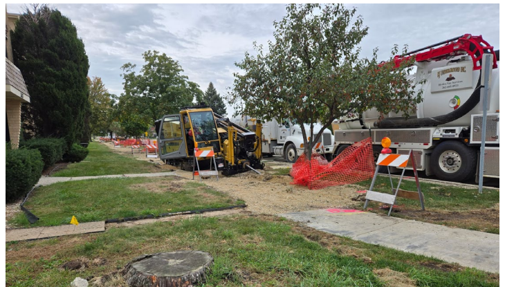
RJ Underground Inc. directional drilling water main on Elm St
